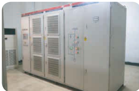
Installing frequency inverter to the slurry circulating pump
