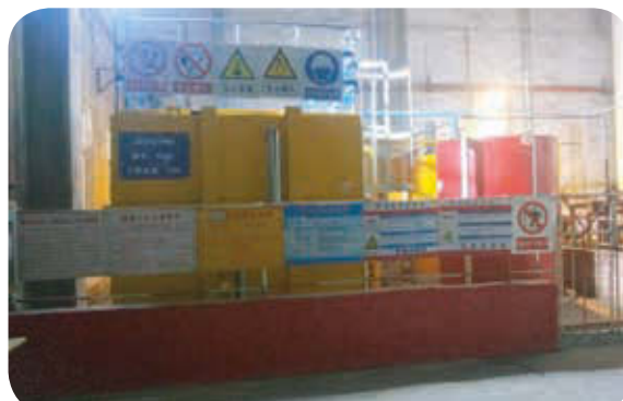
Installing caustic tank and caustic unloading pump to the desulphurisation acid and alkali system
